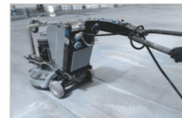
地坪研磨 Floor grinding equipment
