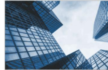
楼宇供水 Building water supply
