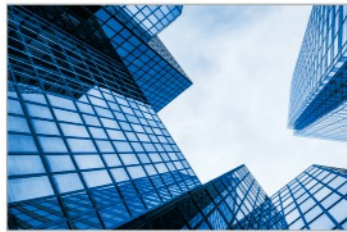
楼宇供水 Building water supply
