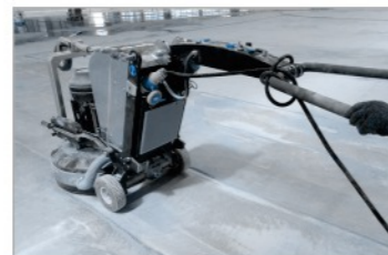
地坪研磨 Floor grinding equipment
